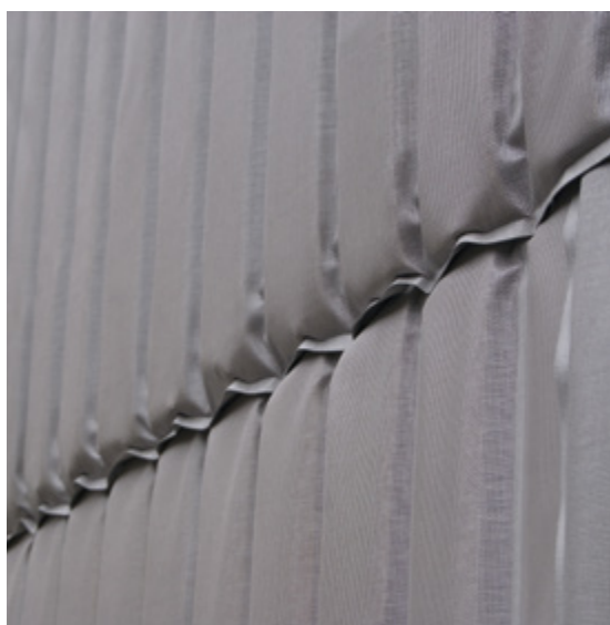
Figura 7: Solapamiento vertical
